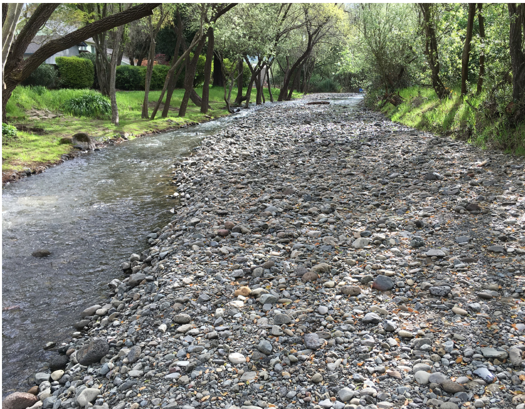
Sediment basin at Snyder Lane where the Sonoma County Water Agency removes coarse grained sediment to prevent flooding in Rohnert Park.
